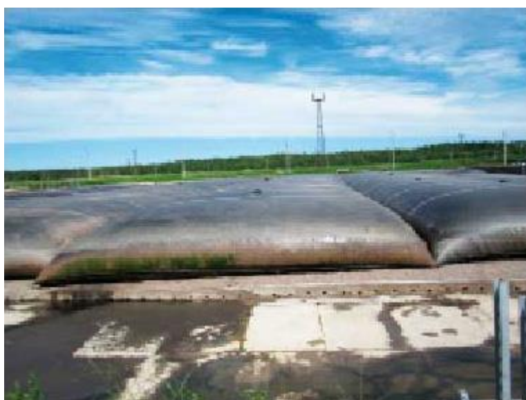
Fig. 10.1. Geotubes filled with recycled wastewater sediment
