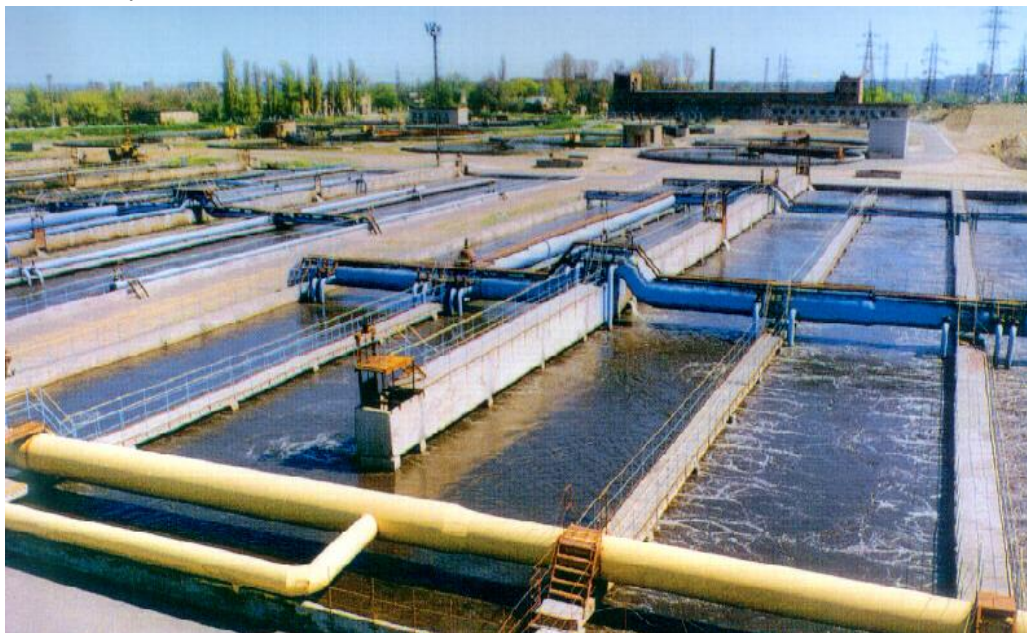
Fig. 3.3. General view of the aeration tank
